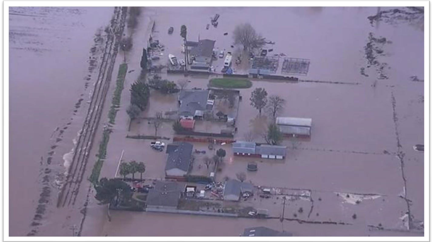
January 11, 2017, Flooding from Pacheco Creek
